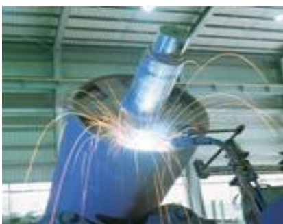
Automatic CO 2 / MIG welding process for End Disk and Shell .
